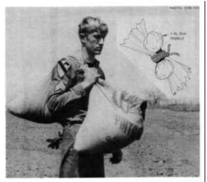
Fig. 8.2. Folding and tying the mouth of a water-filled plastic bag. (Illustration)
