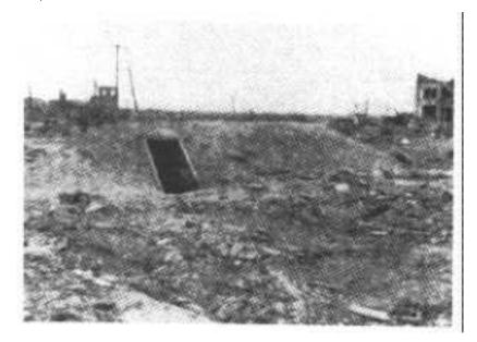
Although the shelter itself was undamaged, its occupants would have been fatally injured because the shelter had no blast door. The combined effect of blast waves, excessive pressure, blast wind, and burns from extremely hot dust blown into the shelter (the popcorning effect) and from the heated air would have killed the occupants. For people to survive in areas of severe blast, their shelters must have strong blast doors.
