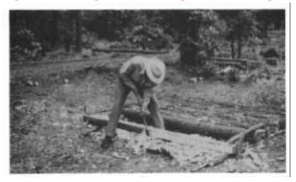
To hew a second flat side at right angles to the first side, rotate the pole 900, secure it again, and repeat as
