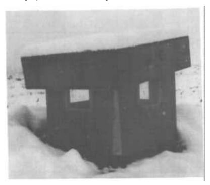
The adjustable top of this exit housing measures  $4 \times 4 \times 1$  feet, and can be tilted to make different sized ventilation openings in any of four directions. The top also can be raised straight up to make various sized openings all the way around, or it can be completely closed - as explained by Fig. F.2 and the following descriptions of its uses.
