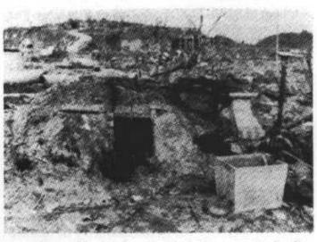
Fig. 1.5. Undamaged earth-covered family shelter in Nagasaki.
